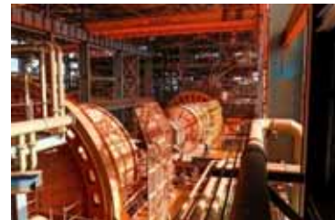
Ball mill and pipeline repairs completed
