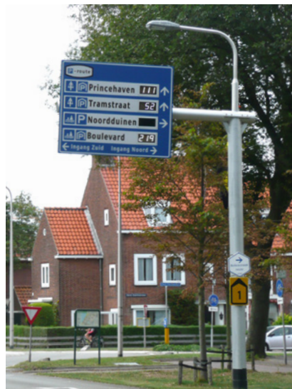
PRIS (parking system) incl. lighting
