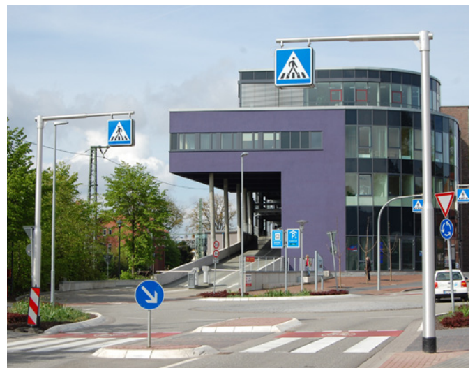
Support for pedestrian crossing sign
