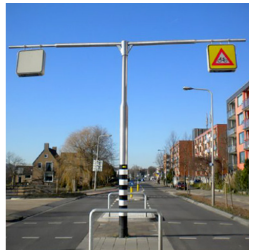
Support for pedestrian crossing sign
