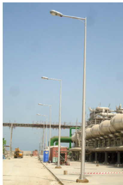
Shuaiba Refinery – Kuwait
