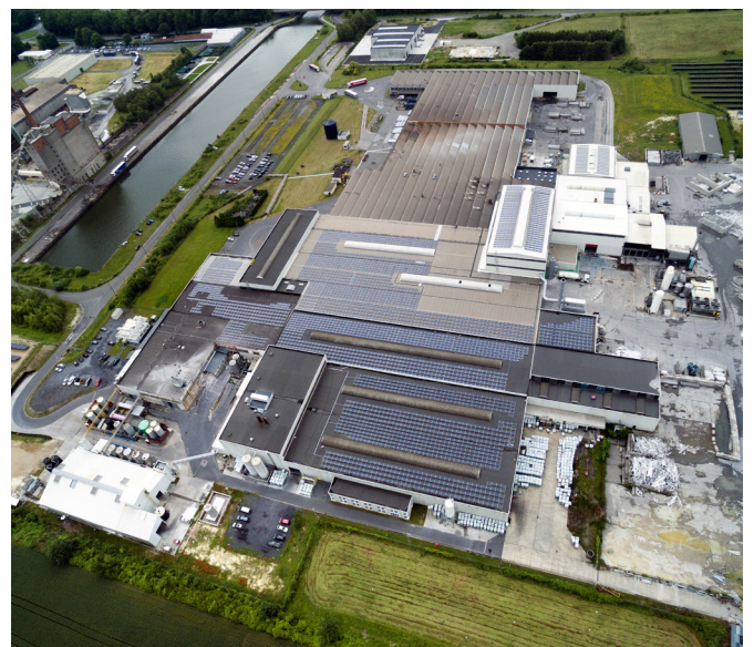
Ghlin casthouse (Belgium)
