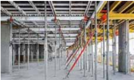
Aluminium formwork for B&C
