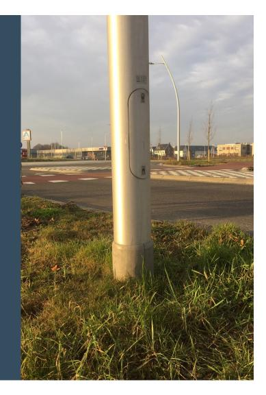
The ground level protector prevents the column from being damaged at ground level, e.g. during mechanical sweeping, mowing or paving activities, or the installation of the column.
