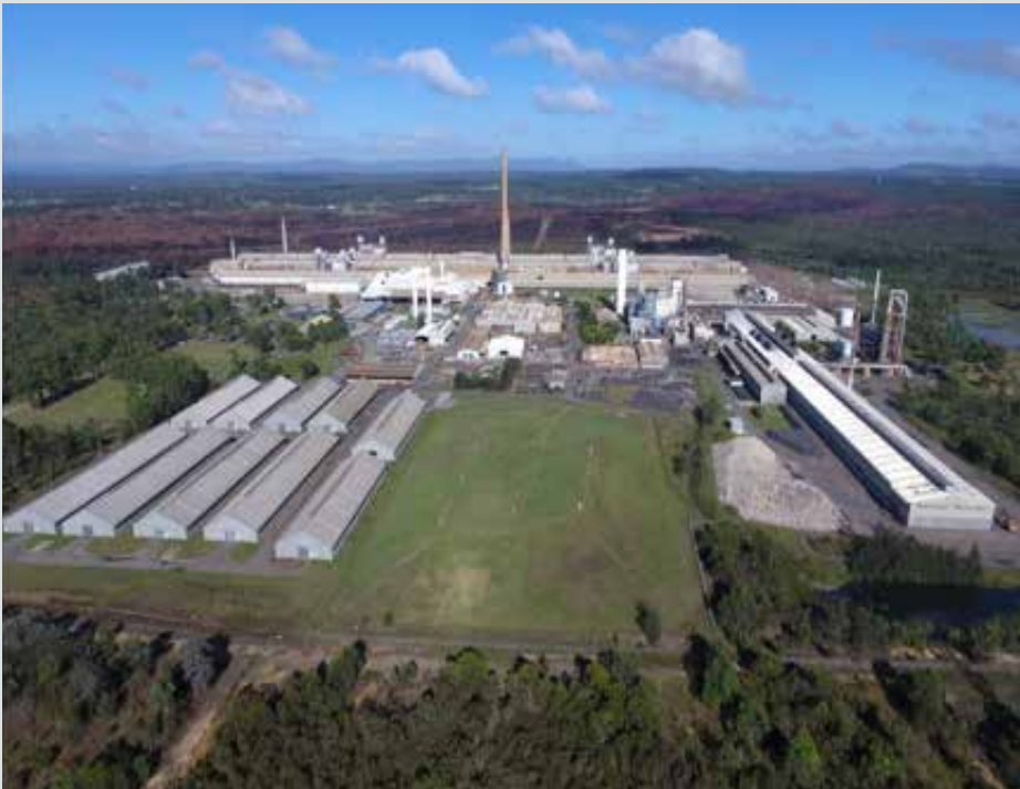
The stacks in this photograph will be demolished as part of Stage 2 demolition, and require an environmental impact statement.
